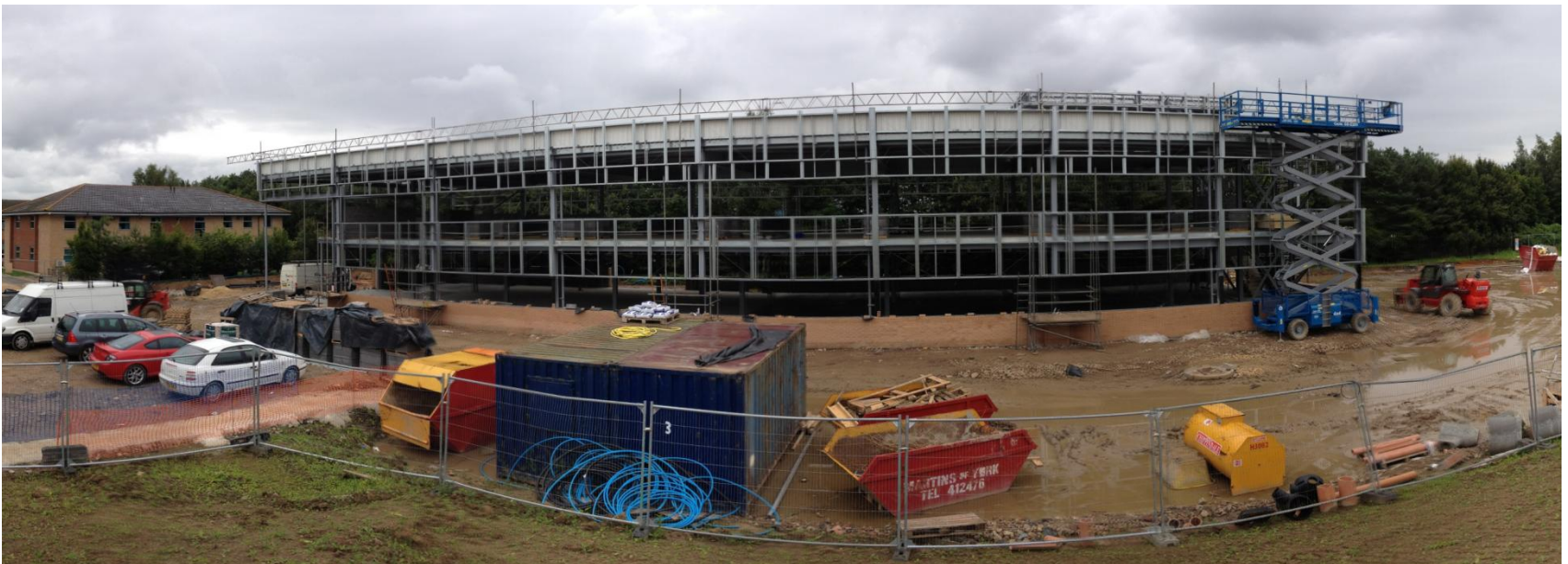
Progress on new MDL building, York
